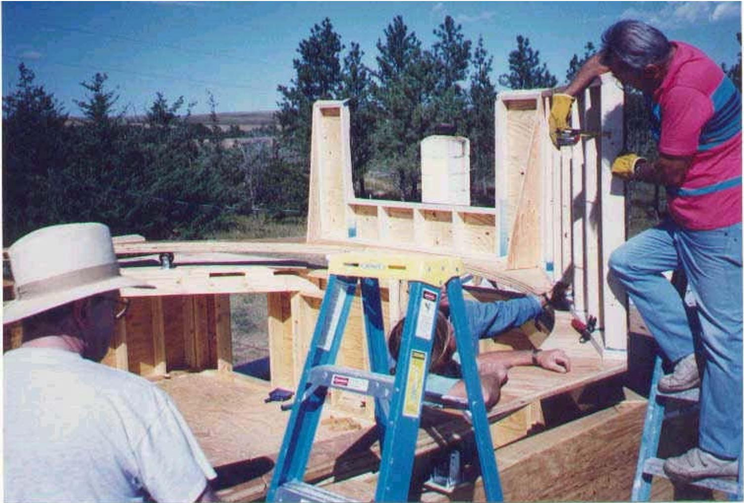
**Dome panels had been constructed ahead of time, and then assembled on site.**
