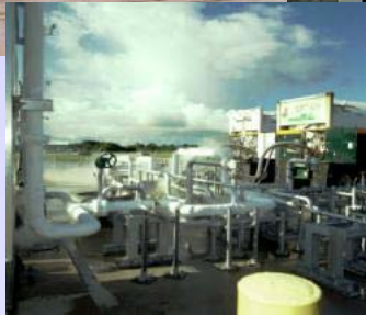
Cryogenic Storage, Distribution, and Servicing Systems
